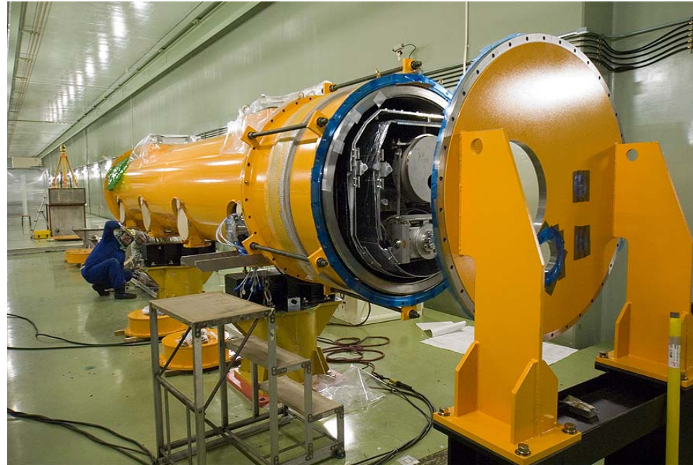
cryomodule sit in the tunnel
