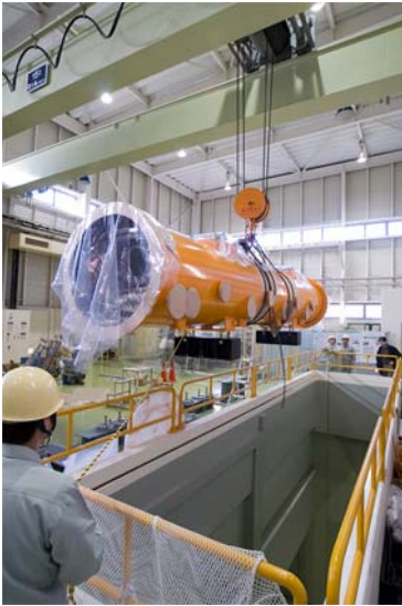
carrying down the cryomodule
