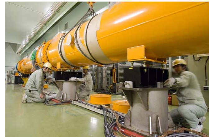
Cryomodule installation
