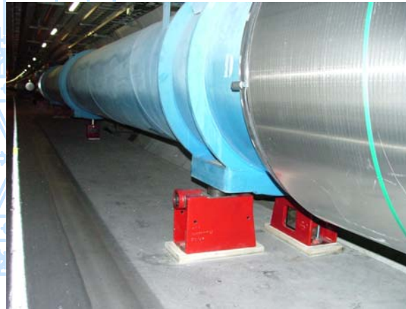
LHC standard cryodipole installed in the 3-4 arc section
