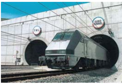
A Eurostar high speed passenger train leaving the EuroTunnel.
