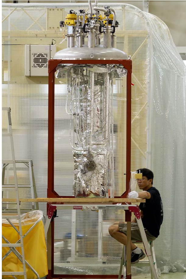
Valve box after repair(8/15)
