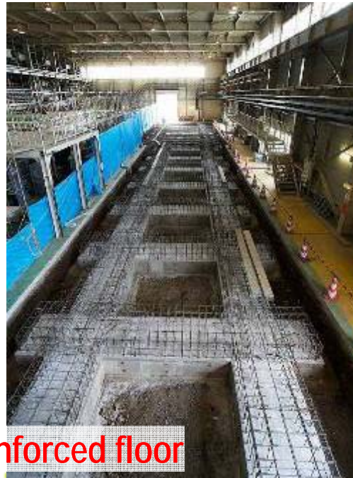
Construction of shielding
