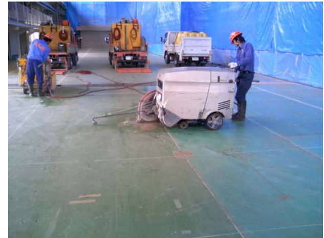
Remove surface concrete 2007/6/27~
