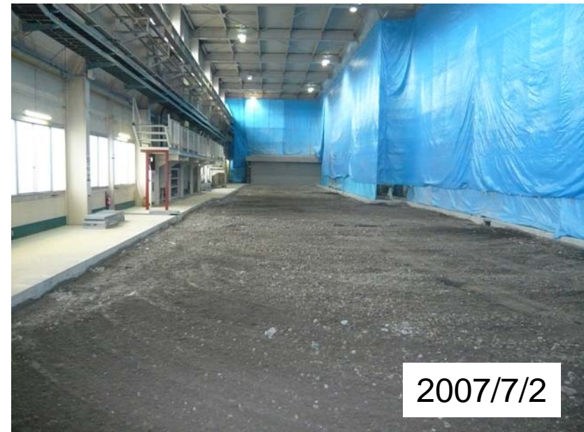
Remove surface concrete 2007/6/27~
