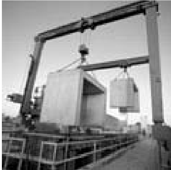
At the precast plant
