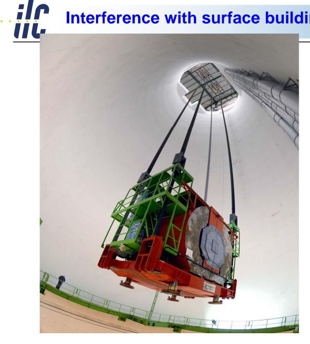
**First heavy lift with** the 350-ton Hadronic Forward **Calorimeters Nov. 06**
