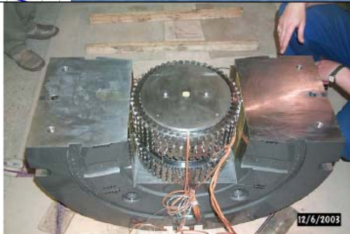
Figure 93 Assembling of pole coils with yoke.
