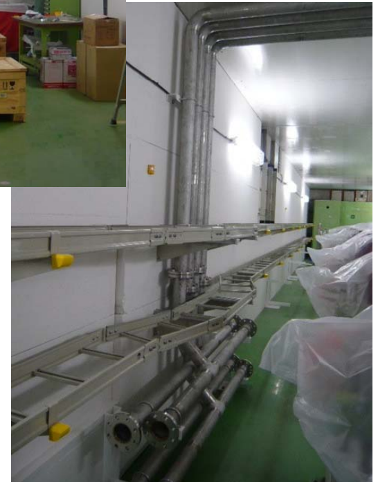
Water piping had been started. (Mar/2008~)
