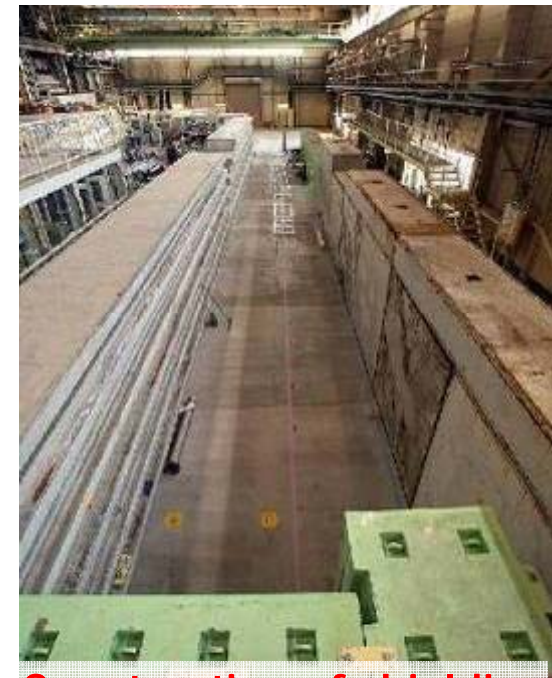
Construction of shielding : 57
