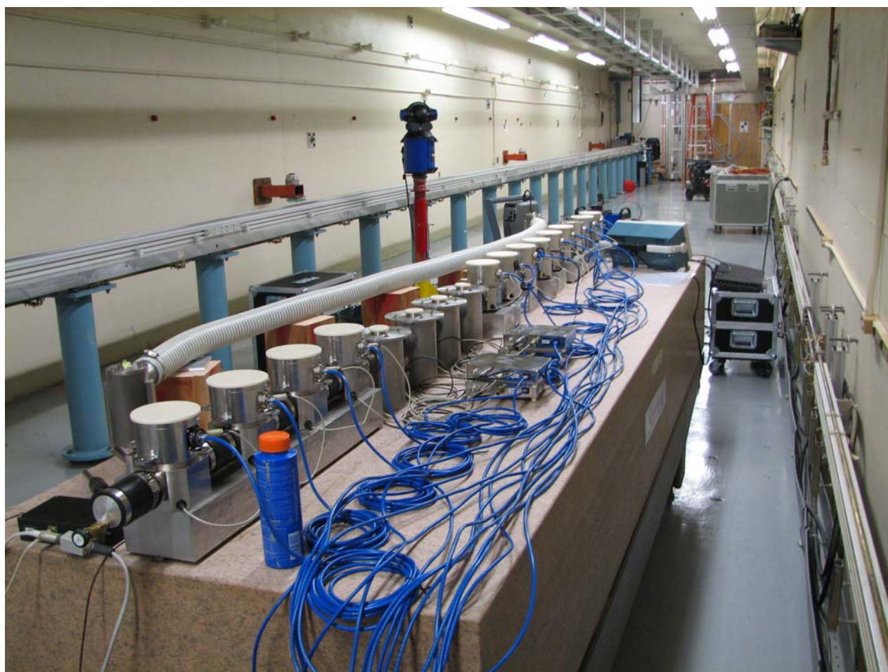
Test stand with pilot patterns of SASE and ULSE at SLAC. May 2006
