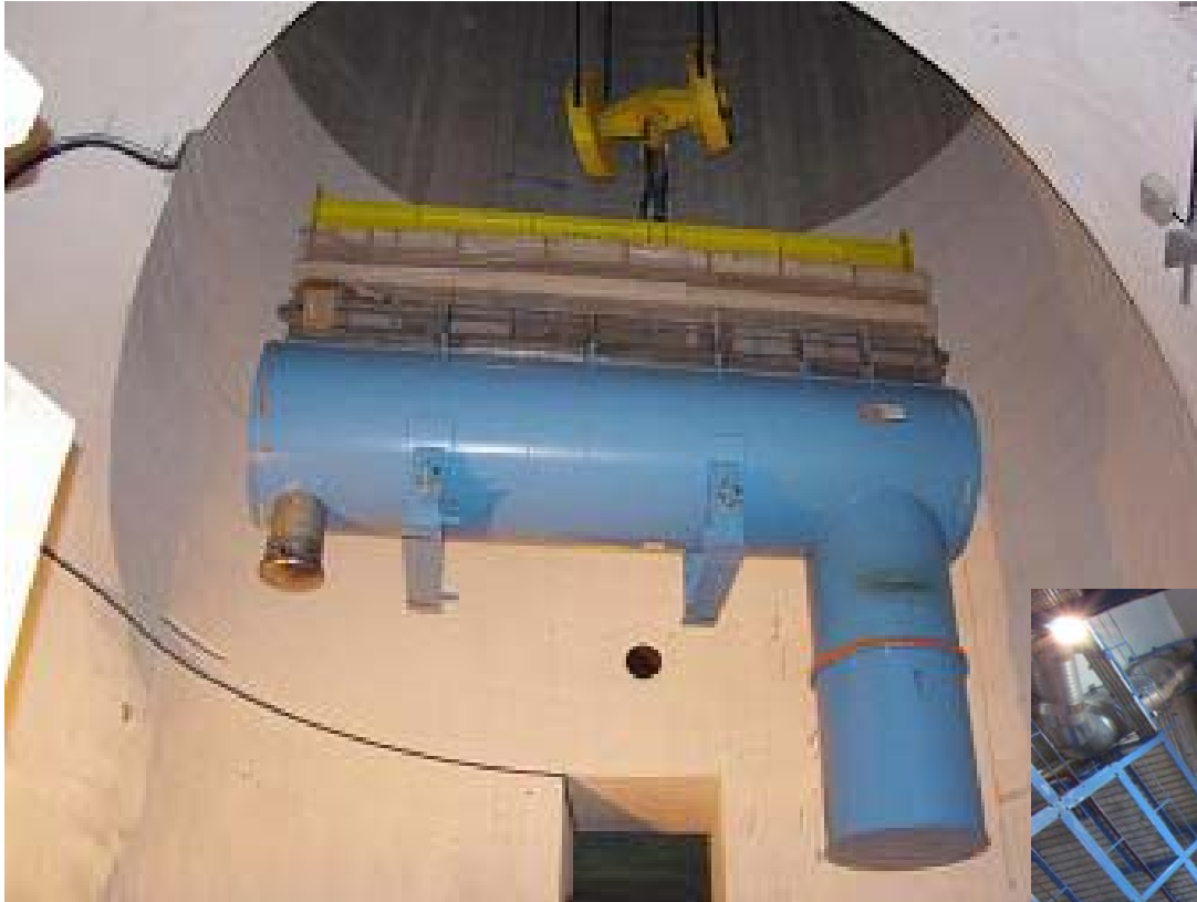
Lower coldbox installation at CERN About 7 m long and 7 m tall, 2 m dia
