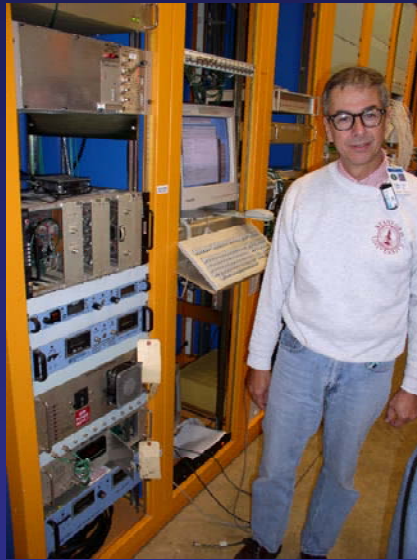
Peter Prieto in front of pulsing circuit for QXR
