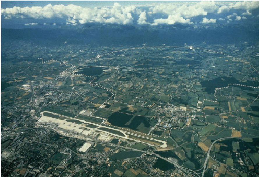
Aerial view of the CERN site with an indication of the circular LEP tunnel
