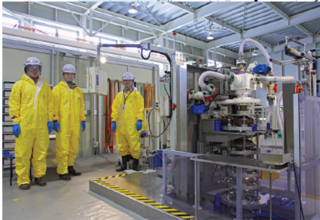
STF – EP system commissioning using old MHI cavity Picture shows acid draining by holding cavity up. 3 times EP cycle (40+60+60 \mu m removal) were done.
