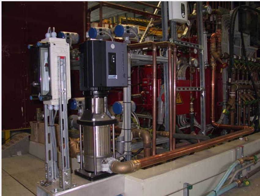
Collector cooling water return bypass
