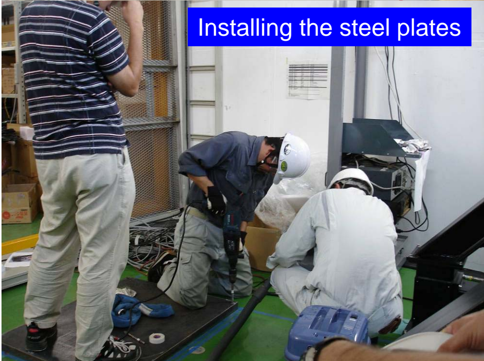
Check height at each step of installation
