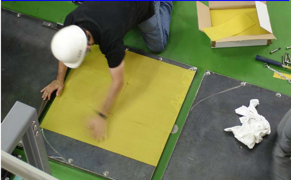
Installing beeswax on plates bolted to the ground
