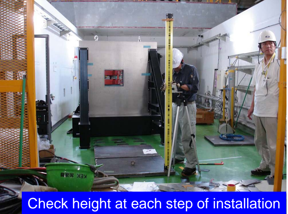
Installing the steel plates
