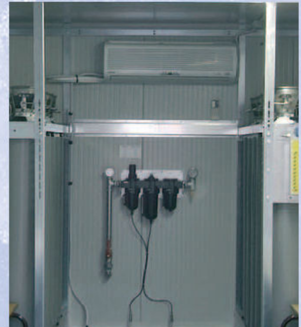
AIR FILTERING SYSTEM
