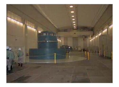
An example of underground facilities constructed in granite geology: Tenryugawa-Sakuma underground dam plant without lining worked more than 50 years without any troubles.
