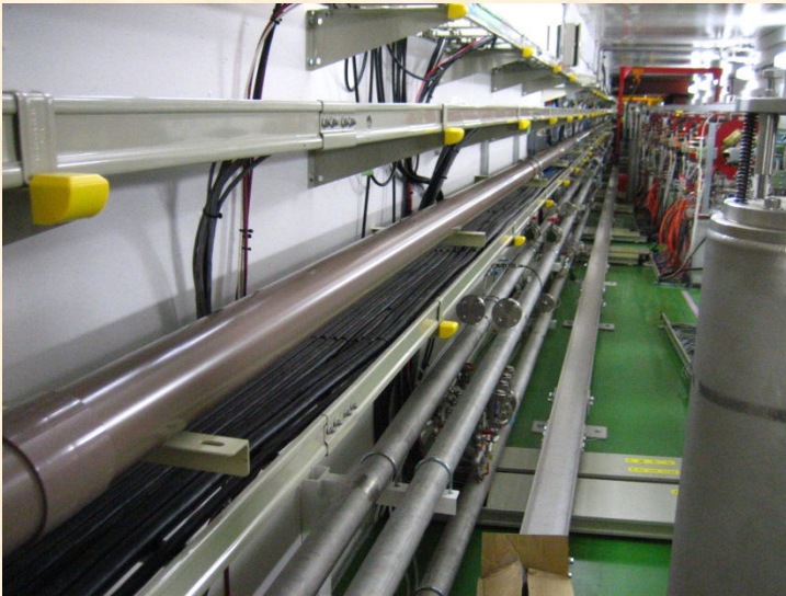
Laser Transport Line (light brown plastic pipe)
