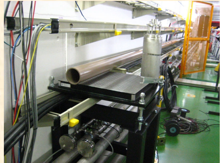
Optical Table for Laser Transport and End of Transport Pipe
