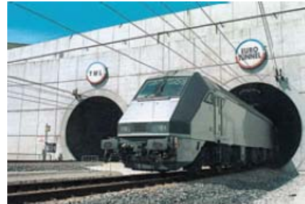
A Eurostar high speed passenger train leaving the EuroTunnel.
