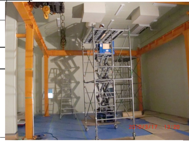
EBW place and crane girder
