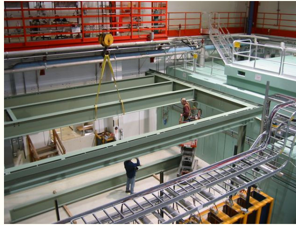
Erection of Laser Deck
