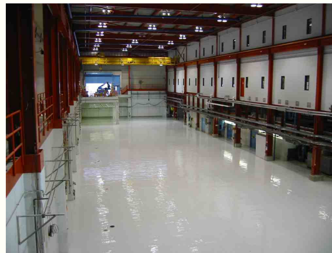
NML Facility after CCM Removal and Floor Painting (February, 2007)
