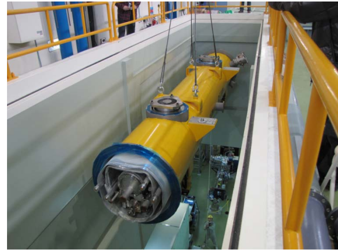
Moving the Module-C into the STF tunnel
