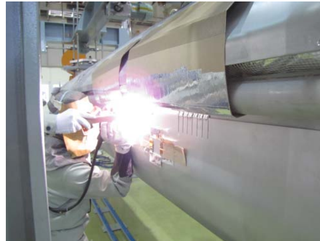
Welding of 5K shield.
