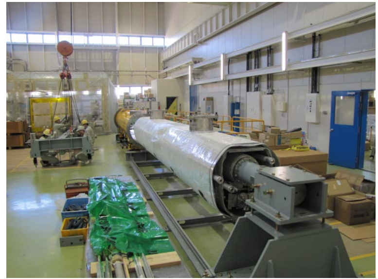
Setting the cold mass on the equipment
