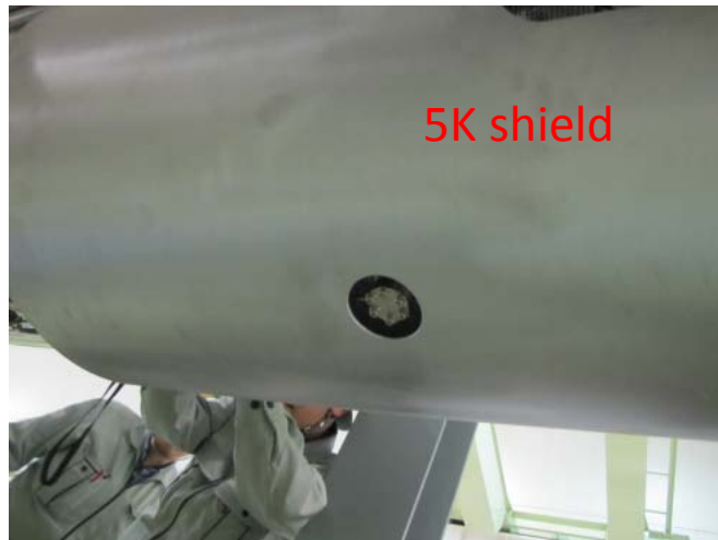
Making holes for FNAL cool-down pipe connection
