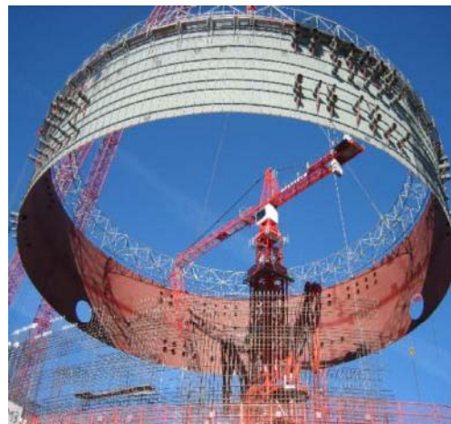
Positioning of a Liner- Segment on EPR Reactor OL 3 Finland
