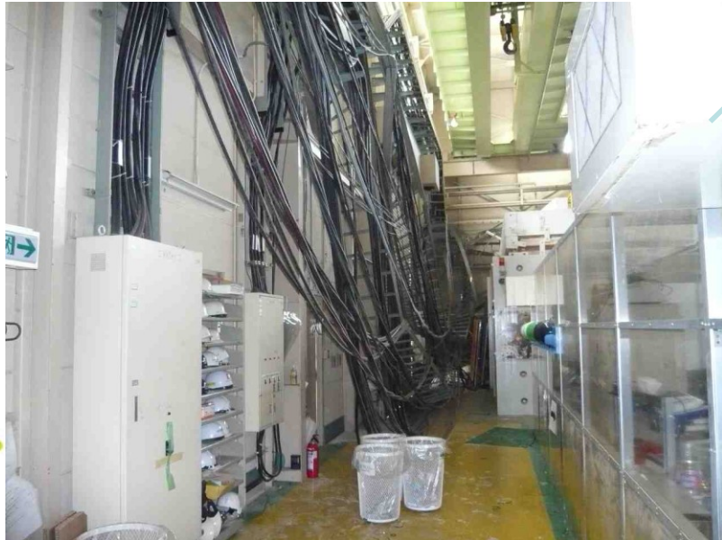
Main power cables for the ATF building
