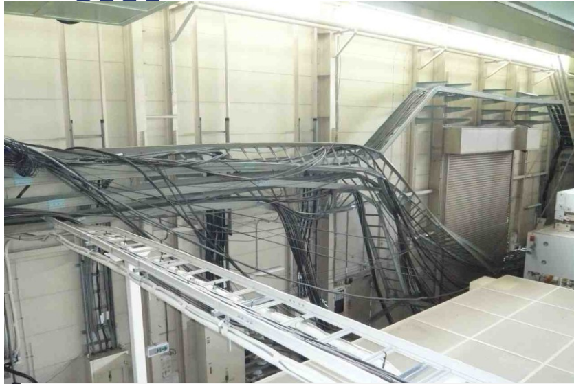
Main power cables for the ATF building
