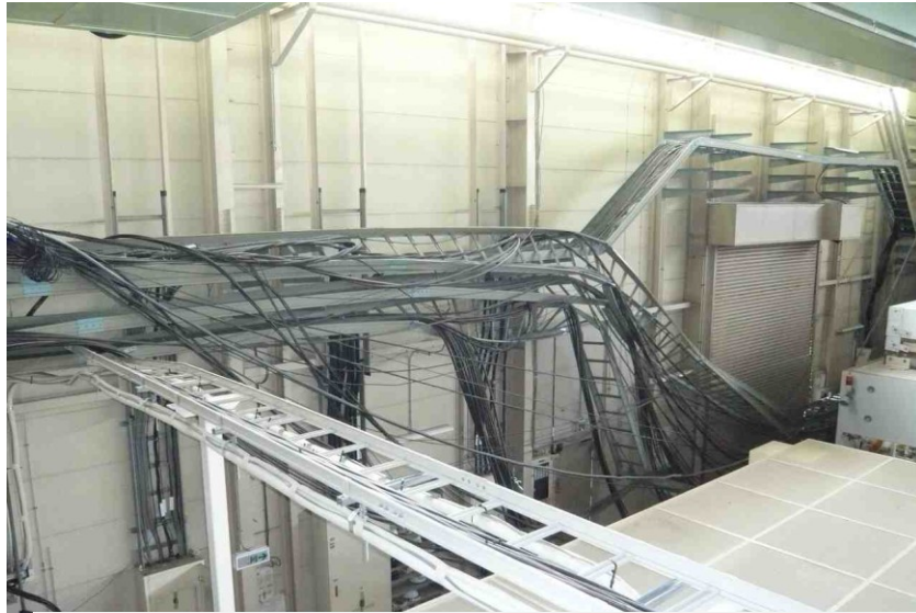
Main power cables for the ATF building
