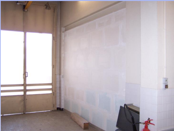
Interior view of Exterior door and wall to 2nd room
