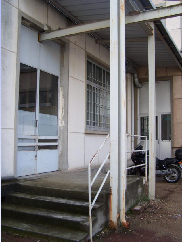
Exterior view of entrance with hoist rail
