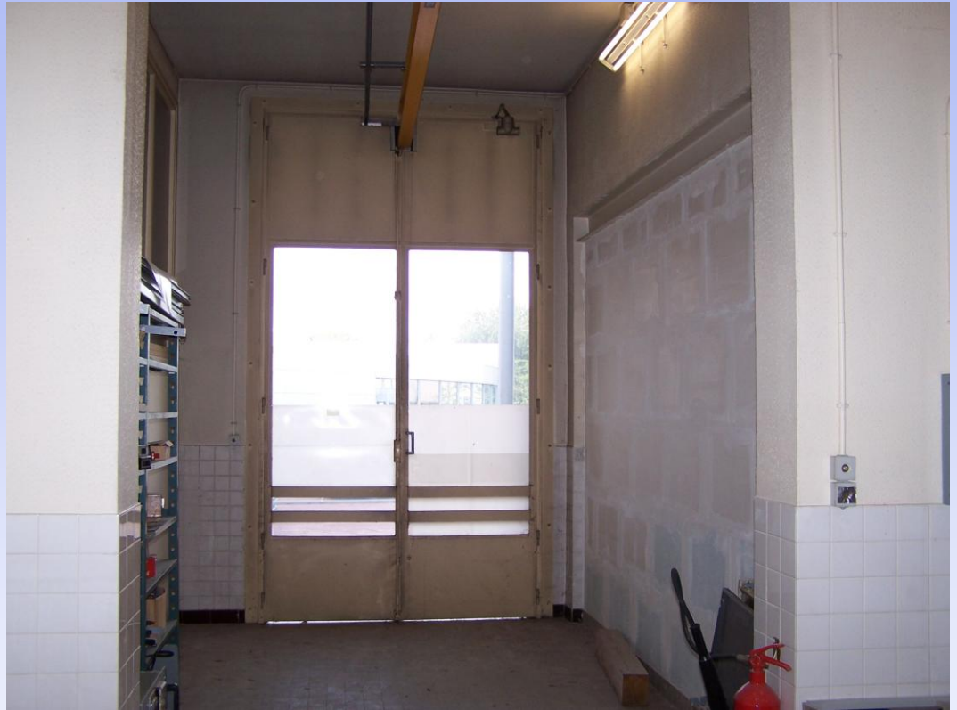
Interior view of Exterior door and hoist rail
