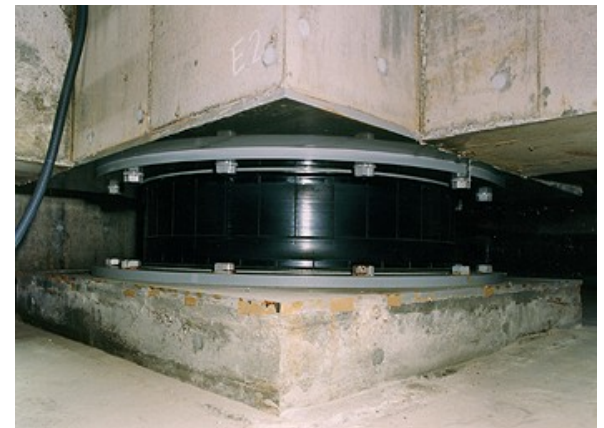
Seismic isolation support for buildings
