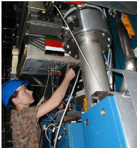
Equipping the front end crates
