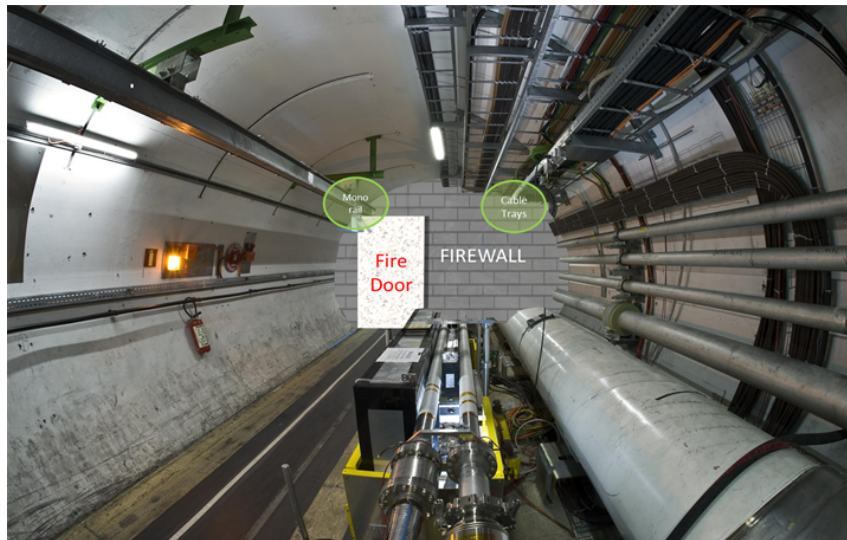
Figure 13.25: Conceptual representation of a firewall transversal to the tunnel orientation
