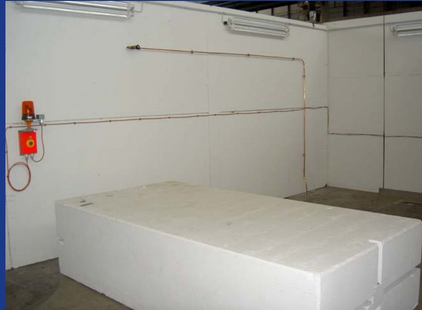
Concrete Block as Base for PCMAG
