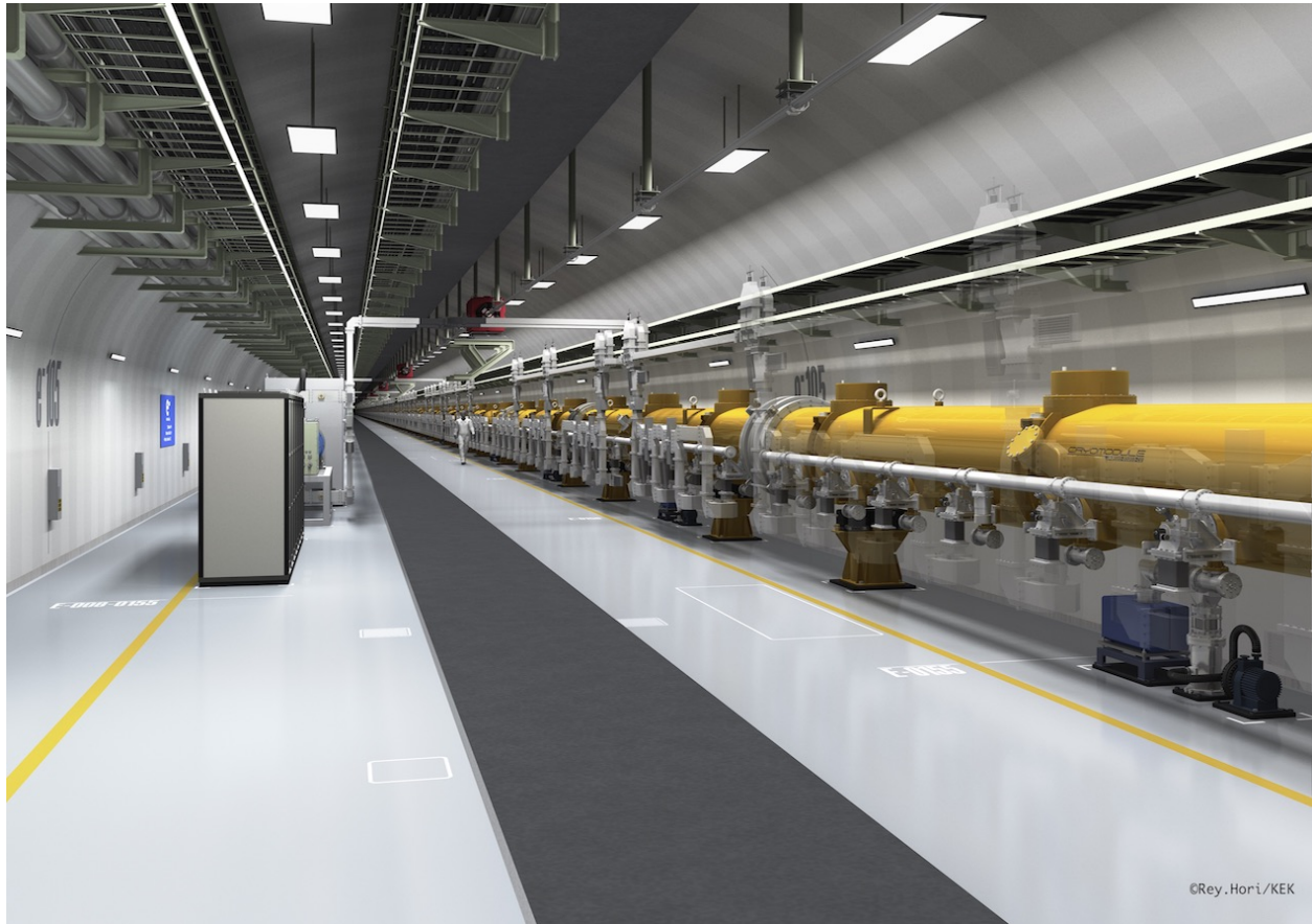
Figure 4.11: Artist's rendition of the ILC Main Linac tunnel. The shield wall in the middle has been removed. ©Rey.Hori/KEK.
