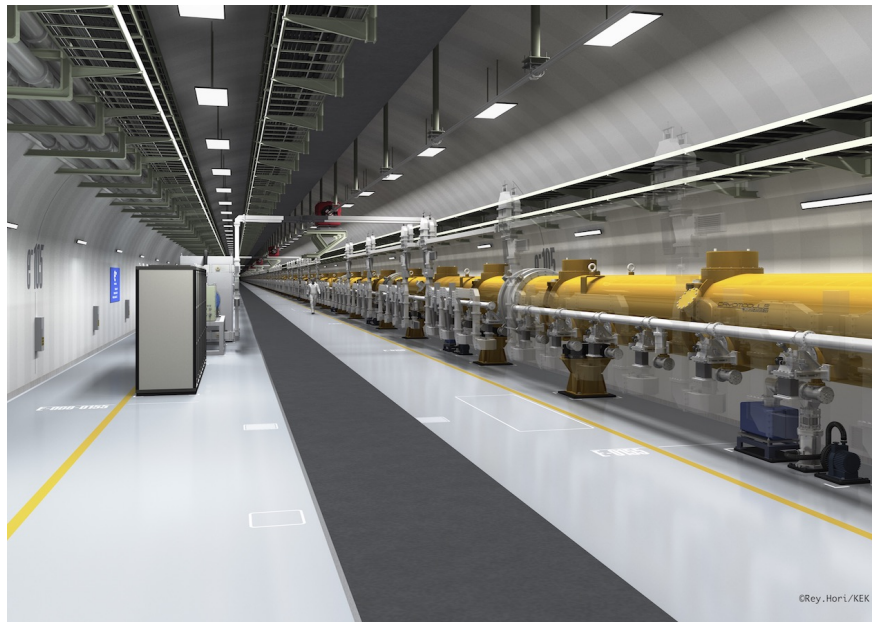
Figure 4.10: Artist's rendition of the ILC Main Linac tunnel. The shield wall in the middle has been removed. ©Rey.Hori/KEK.
