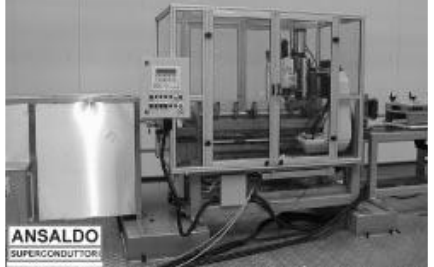
Milling machine, placed aside the cleaning unit : Removing Al-alloy to prepare electric joint at the beginning and at the end
