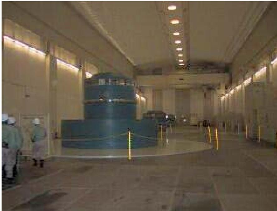
*An example of underground facilities constructed in granite geology: Tenryugawa-Sakuma underground dam plant without lining worked more than 50 years without any troubles.*
