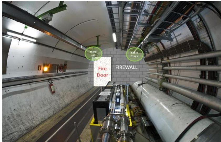
Figure 1- Conceptual representation of a firewall transversal to the tunnel orientation
