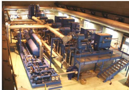
Figure 3 Compressor station of 18 kW @ 4.5 K cryogenic refrigerator
