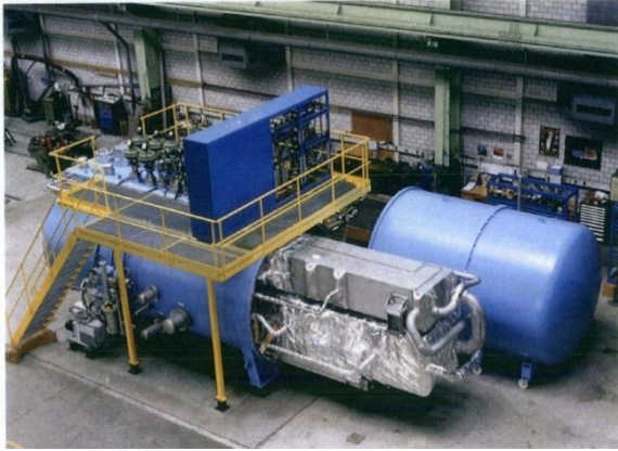
18kW Helium ref. cold box / CERN LHC
