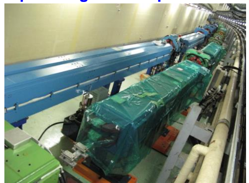
TiN coated beam pipe with antechambers
