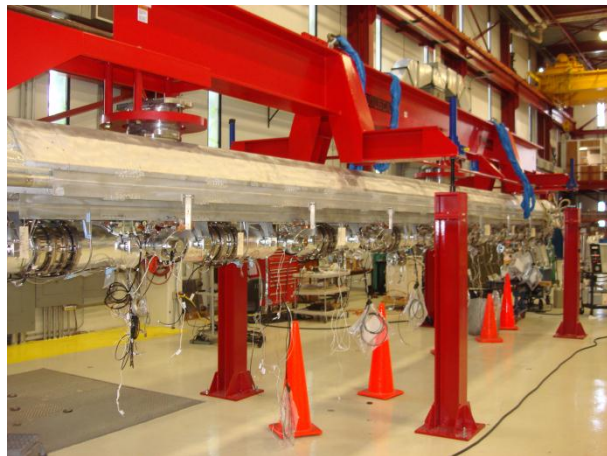
CM2 cold mass was partially disassembled to repair the leak
