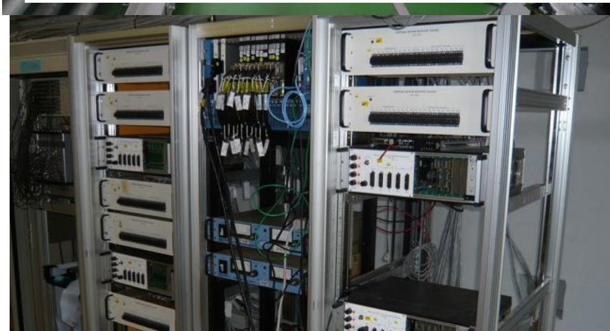
Magnet mover system and QBPM readout (SLAC)
