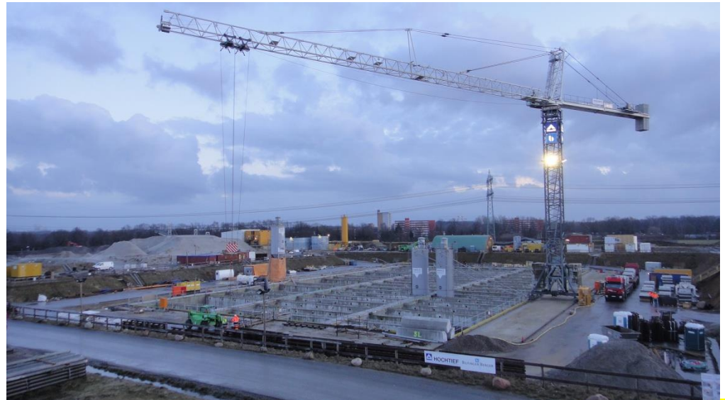
Construction of experimental halls is ongoing.
