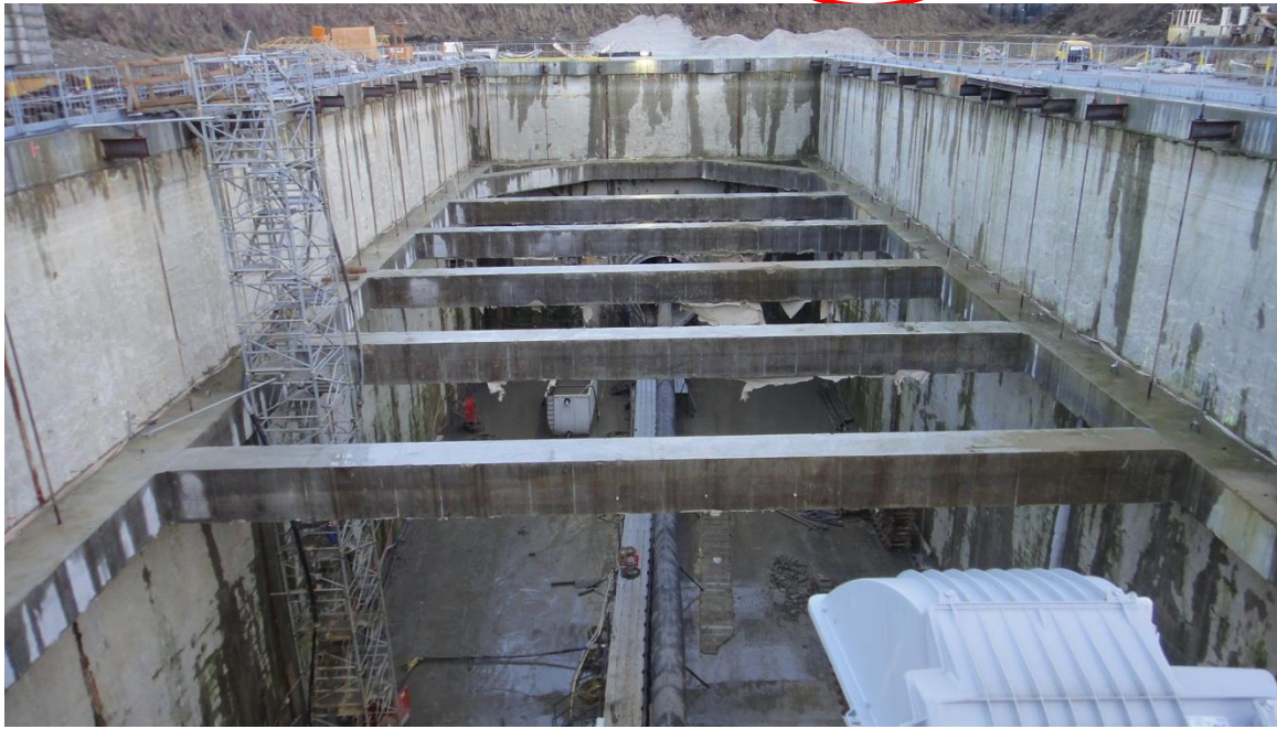
End of SRF linac. Entrance of tunnel boring machines.
